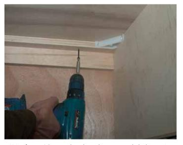
4. Using four 1 1/4" course thread wood screws, attach the base unit to the top by screwing up through the mounting strip into the top. Be careful not to countersink the screws too far.
