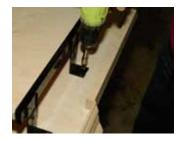
4. Attach the keyboard slide to the desktop using the supplied 1/2" screws.
